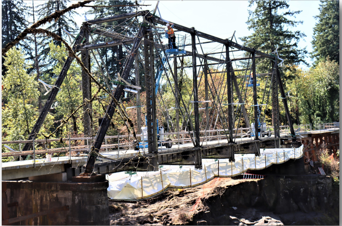
Above: Staff from FD Thomas Painting install debris containment materials on the Mill City pedestrian bridge.
