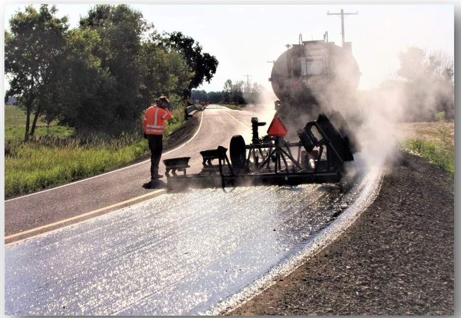
Road Department workers chip seal Bell Plain Road in June.
