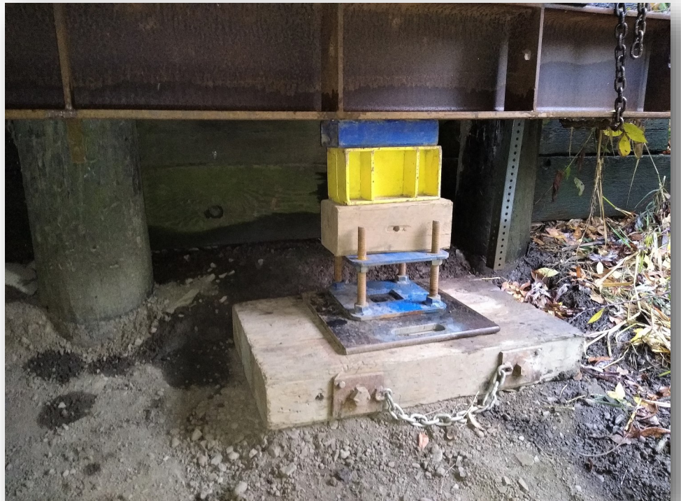
Right: Temporary cap installation on a bridge on Glass Drive.
