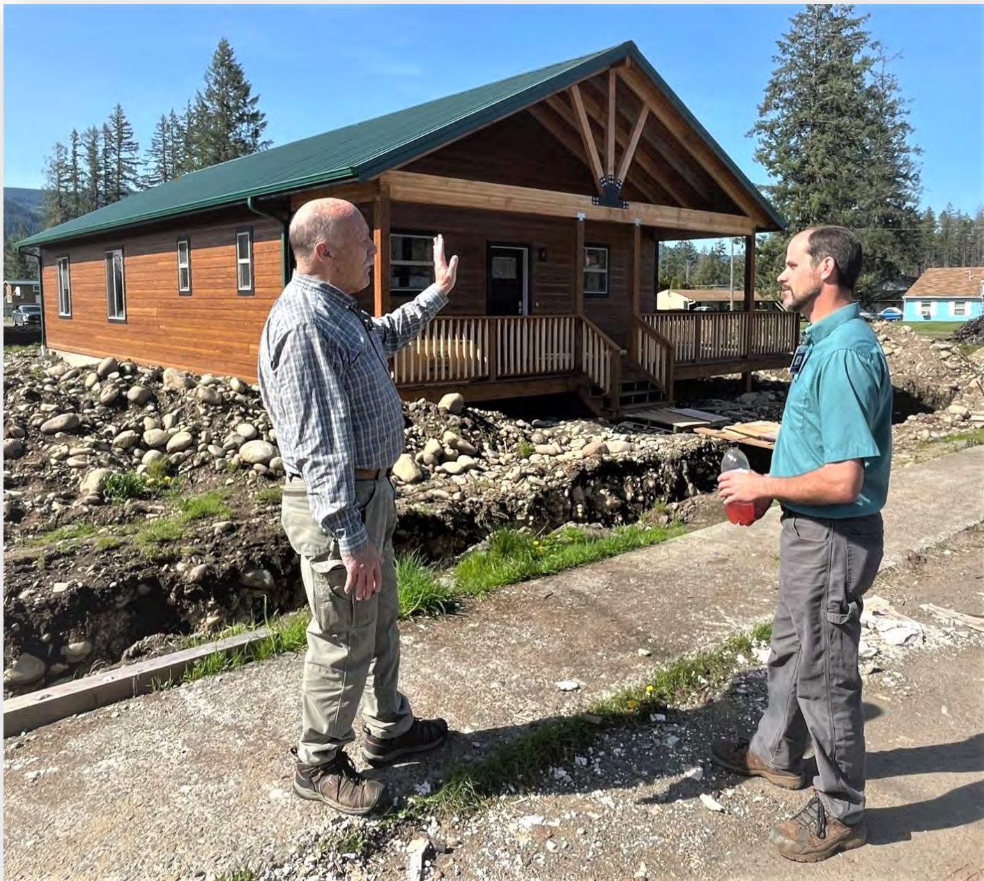
Linn County Commissioner Will Tucker, left, talks with project coordinator Joe Nicholes of Christian Aid Ministries in front of one of 17 new homes that have been constructed in the Santiam Canyon since 2021. Volunteer teams will build 10 more homes starting this Fall.
